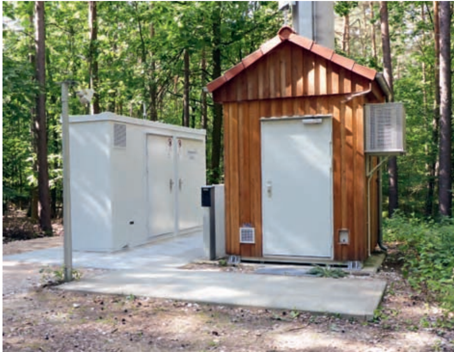
Digital radio base station locations with fuel cell emergency power systems in Bavaria.
