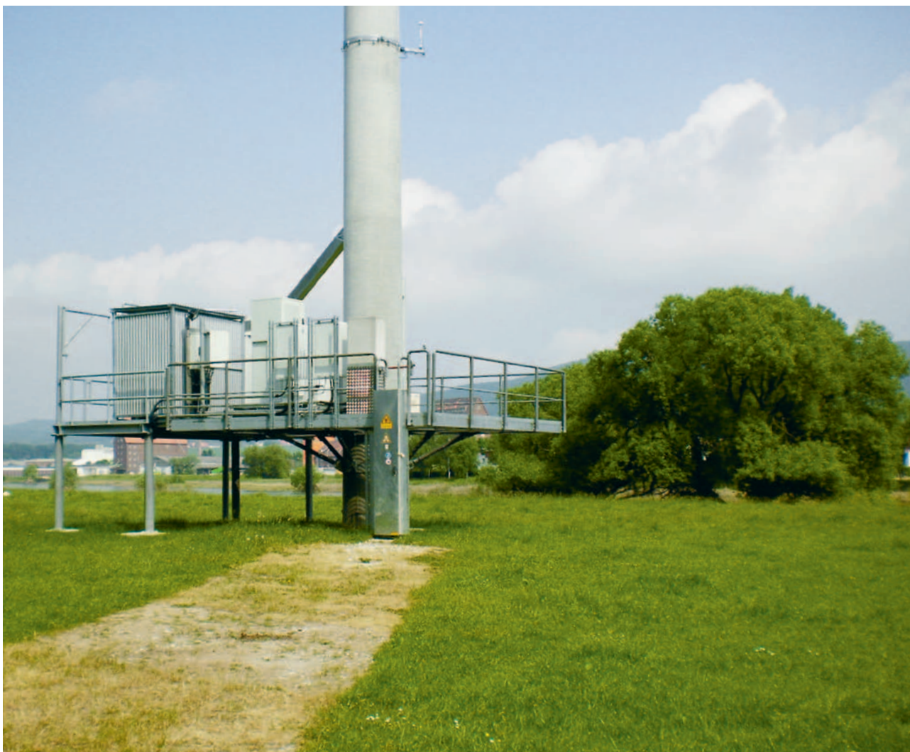
BOS (emergency services) base station fuel cell system
