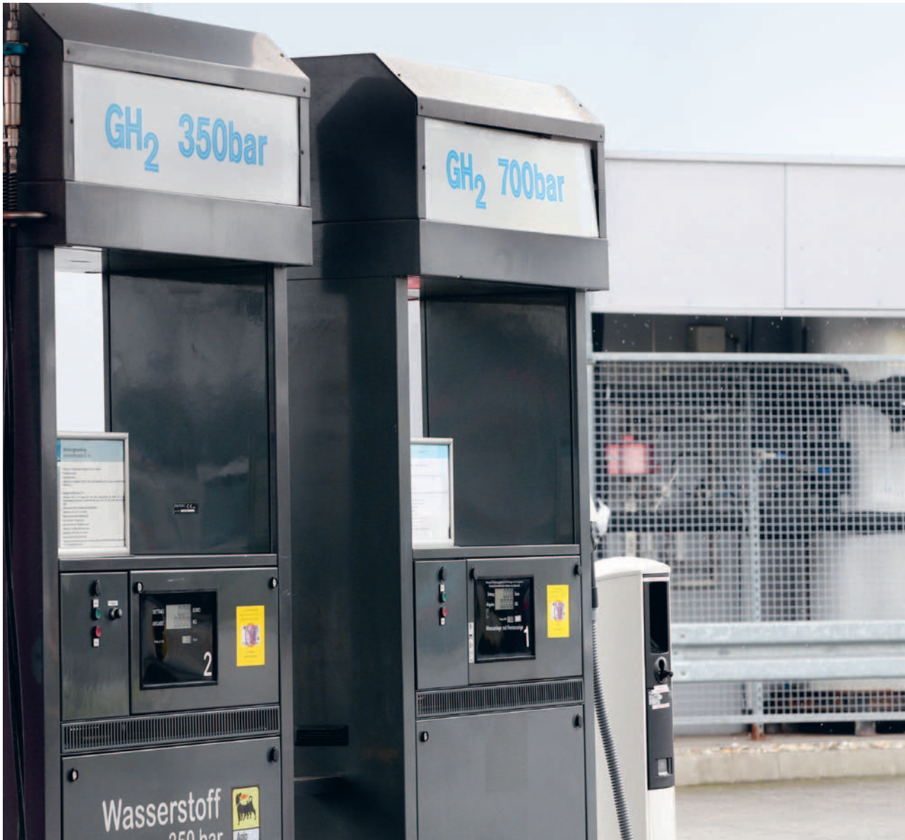
Both fuel cell buses (350 bar) and cars (700 bar) can be refuelled at the hydrogen filling station located in close proximity to Höchst Industrial Park.
